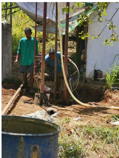
Additional drilling of deep well
